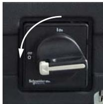
For Bolt On Track, turn off the power switch on the side of the Bolt Base.
