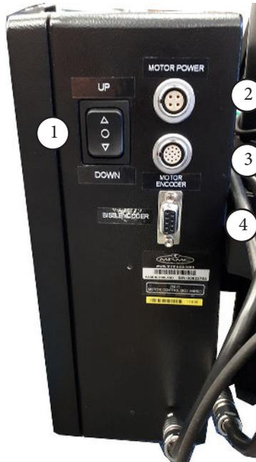
1. **Rocker switch** to move the SLH lift column up or down.
